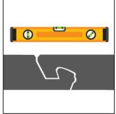
Then carefully knock into place using an acrylic hammer. This makes installation easier and ensures that the front-end connection is locked completely and accurately. Make sure that the panels are absolutely flush with each other.
